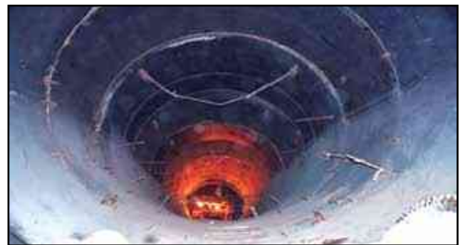
Pressure Shaft & TRC
