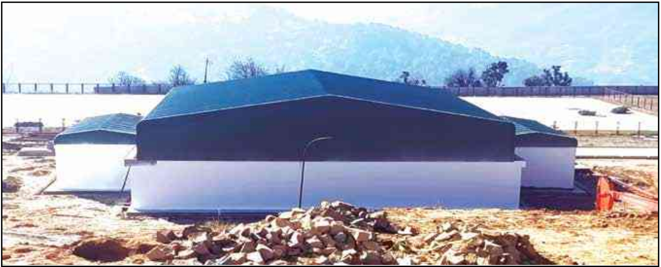
Heliport and Helicopter Shelter
