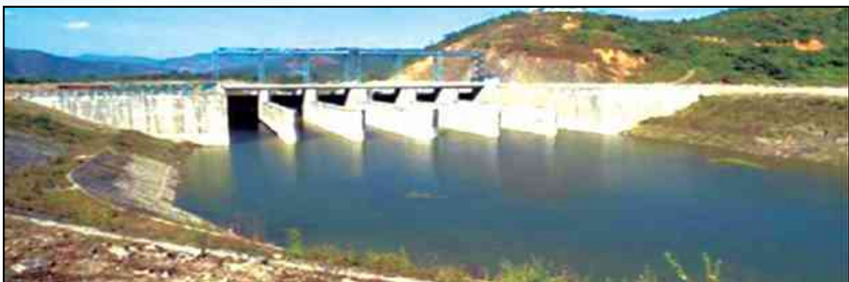
Dolaithabi Barrage, Manipur
