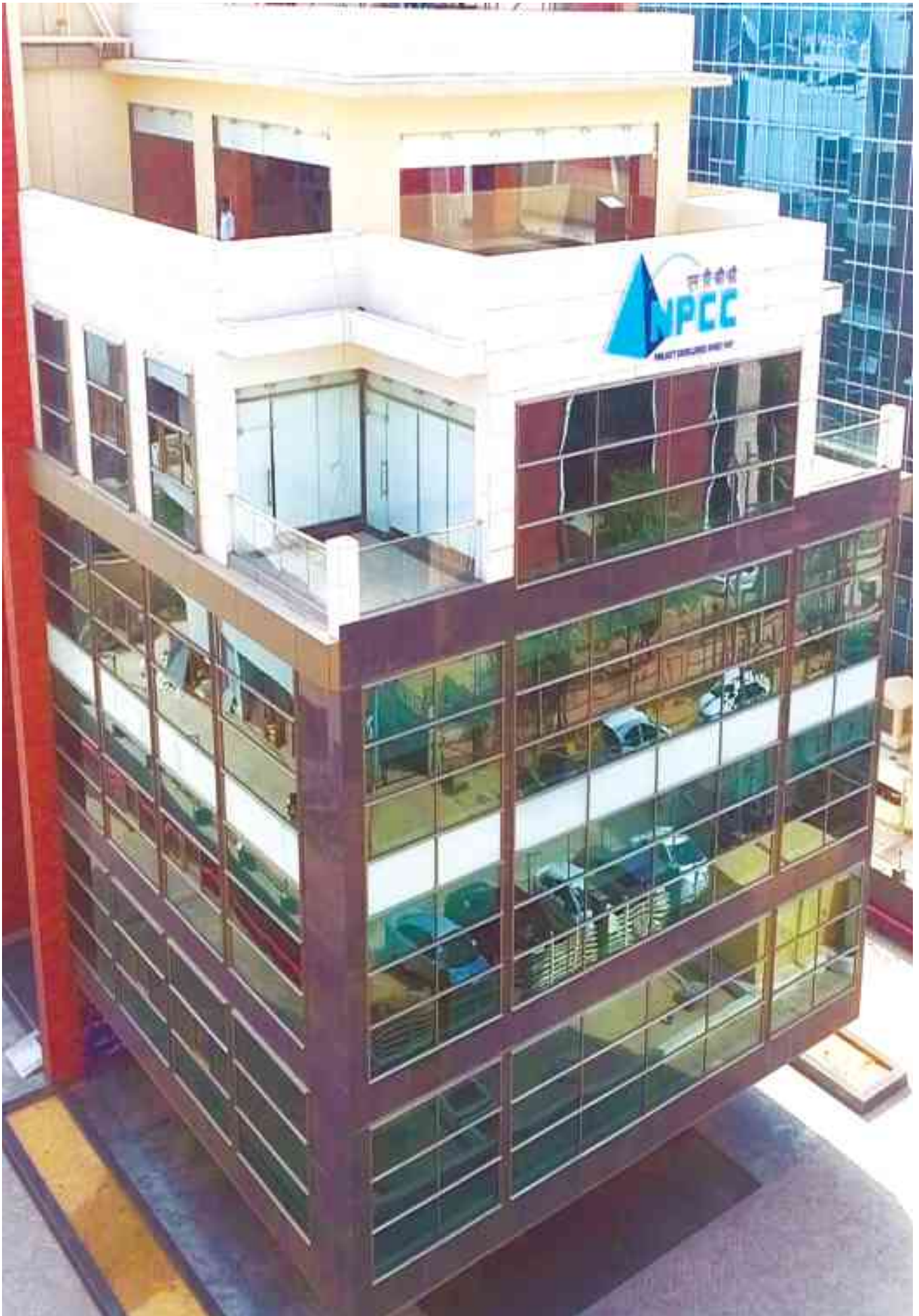
Corporate Office Building, Gurugram
