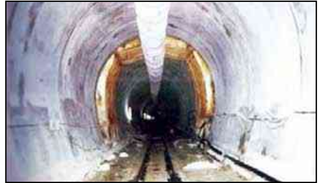
Head Race Tunnel
